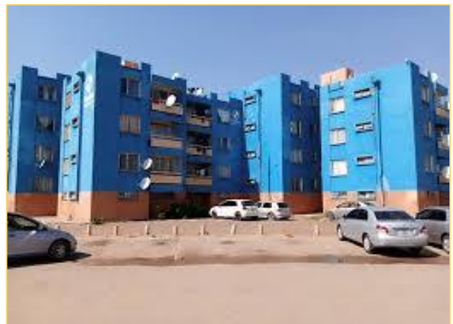
Figure 12: Kabwata Estate Flats in Lusaka
