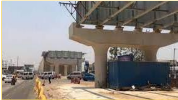
Figure 9: Construction of the flyover bridge in Lusaka
