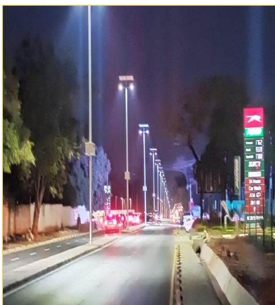
Figure 22: Constructed Roads with street lights in Lusaka
